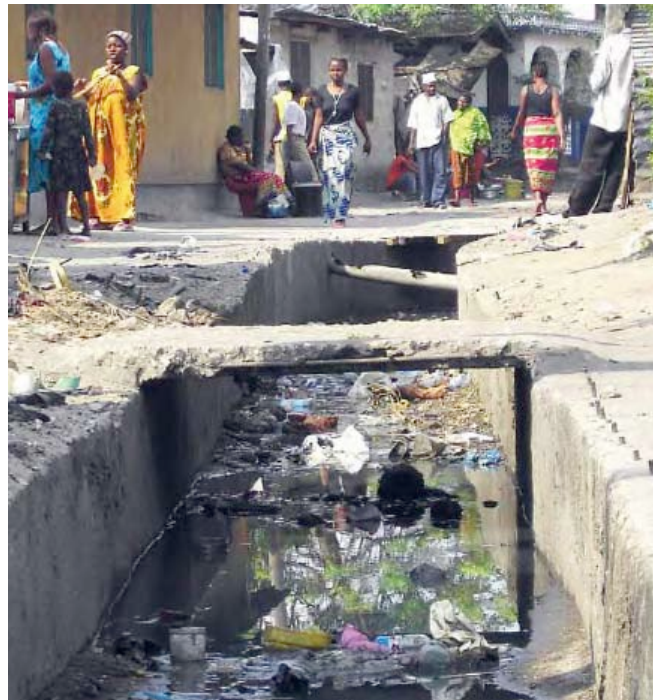
Photo 5: Open drainage in Hanna Nassif, constructed during community-based settlement upgrading
